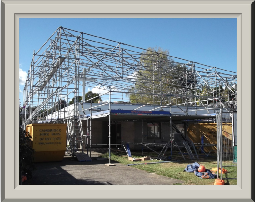
The scaffolding is up for the Baptist Church building.
